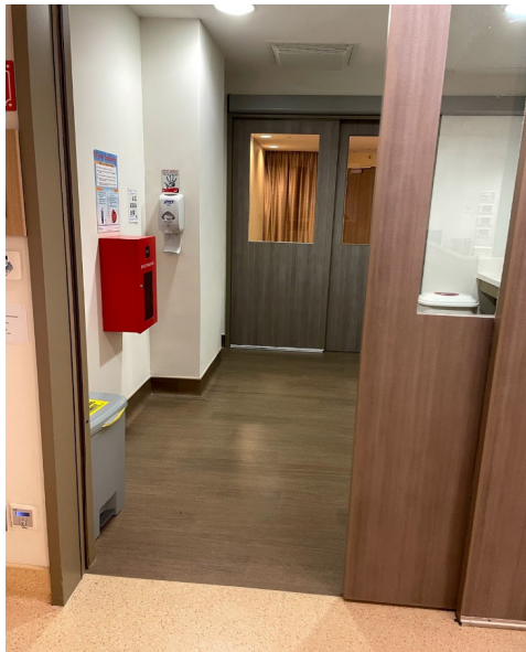
Figure 2: Double doors to maintain negative pressure.
